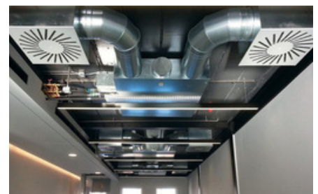
Ducted Air Conditioning Systems These systems use ductwork to distribute cool air throughout a building and are commonly used in larger commercial spaces.
