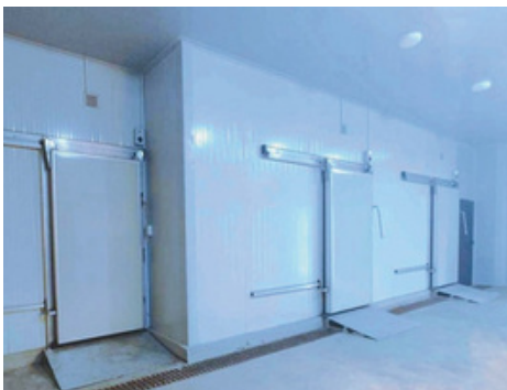
Cold Storage Warehouses
